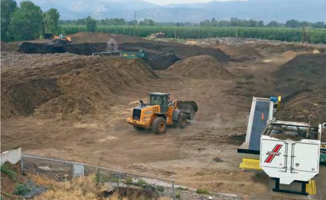
920-18 Stationary Rotary Mixer (920 cu. ft. capacity) Land fill composting operation
